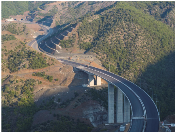
Figure 1. Structures on the Demir Kapija – Smokvica highway (construction phase)
