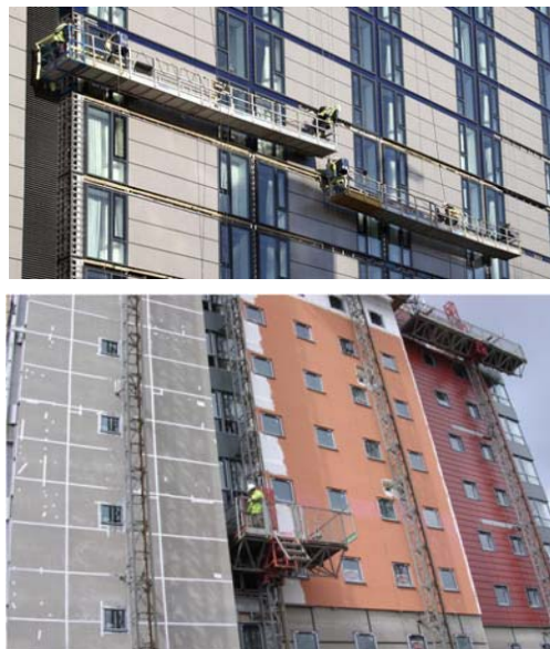
Figure 5. Suspended scaffolding and work-at-height platform (platform moving along a scaffold column) [7-11]
