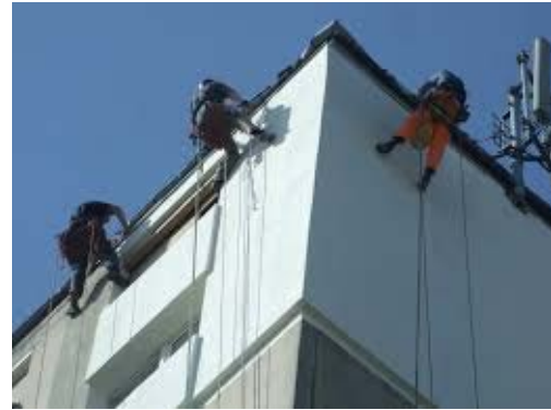
Figure 7. Use of safety belts/harnesses and ropes during roofing and façade work [7-11]
