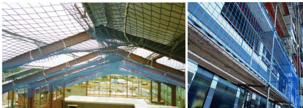
Figure 3. Fall arrest safety net [7-11]
