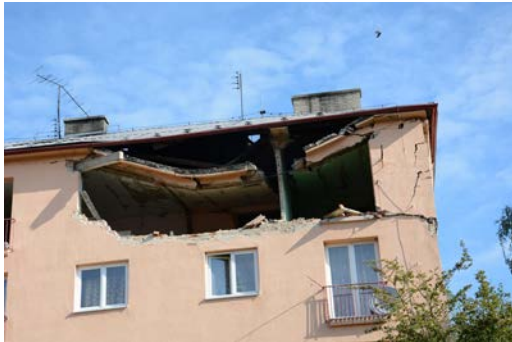
Figure 3. The damaged block of flats after the gas explosion in Havířov [1]
