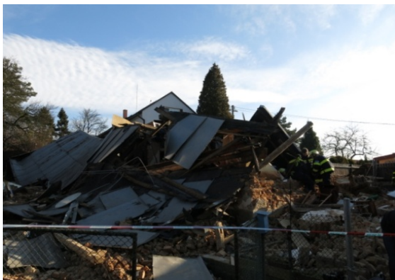
Figure 4. The ruins of the detached house destroyed by a gas explosion [1]
