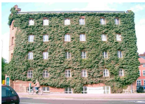
Figure 6. Vertical greening system about 100 years old, Germany [4]
