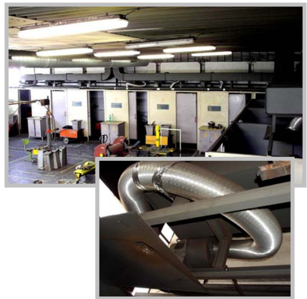
Figure 1. Exhaust system in the welding school
