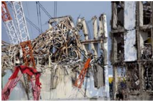
Figure 1. The roof of Unit 3 demolished by hydrogen explosion (left part) and Unit 4 damaged by this explosion (right part). The photo was taken on 28.02.2012.
