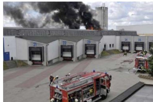
Figure 2. First case - fire begins from photovoltaic modules
