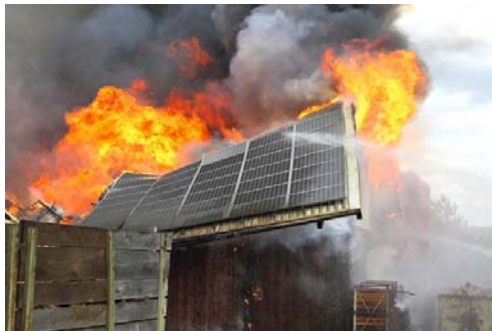
Figure 1. Fire in building integrated photovoltaic systems
