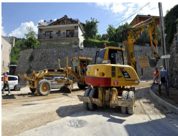
Figure 5. Construction site noise [1]
