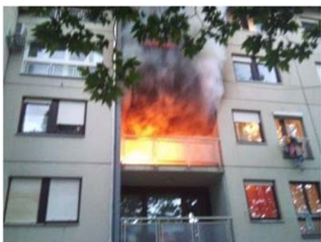
Figure 2. Fire spreading to the floor above
