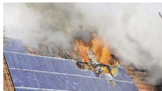
Figure 3. Second case - fire begins from inside the building and covers the roof installation
