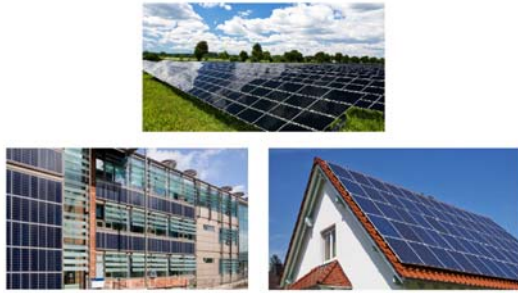
Figure 3. Ground, facade and roof photovoltaic systems
