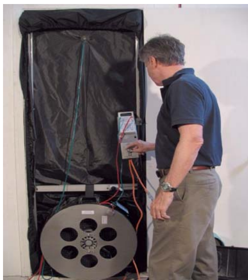
Figure 7. Plate on the door
