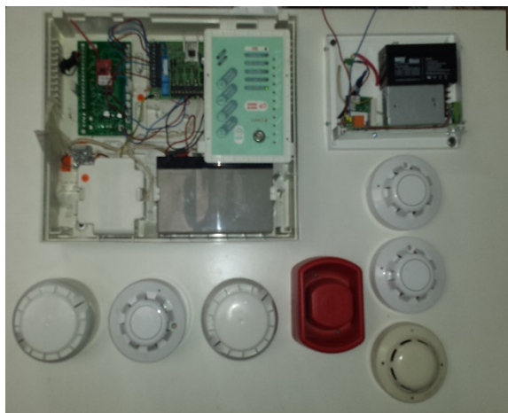
Figure 7. Fire alarm installation
