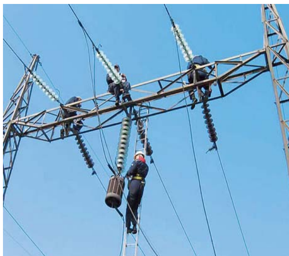
Figure 2. Electrician job performance
