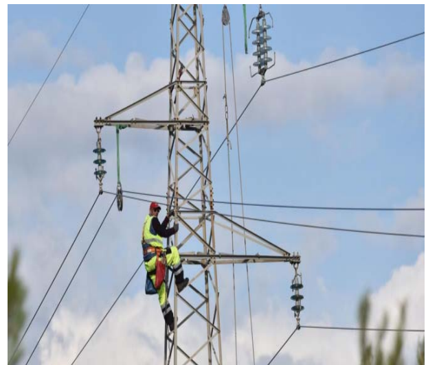
Figure 1. Working at height
